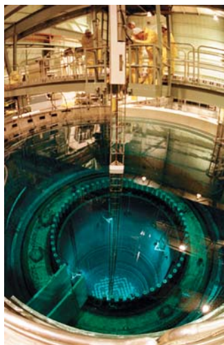
Figure 23.11 Refueling the core of a nuclear reactor.
