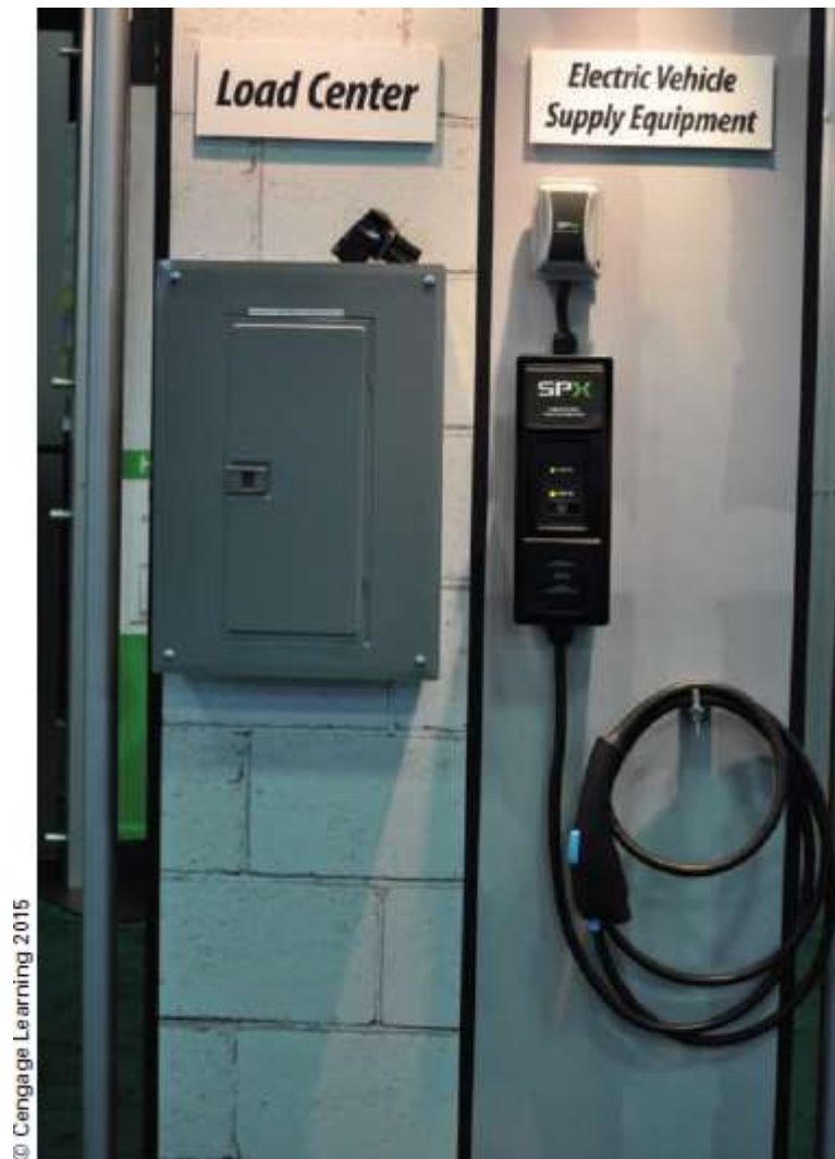
Figure 36-10 An on-the-wall charging unit with a special circuit box (load center) installed to handle the high voltage.
