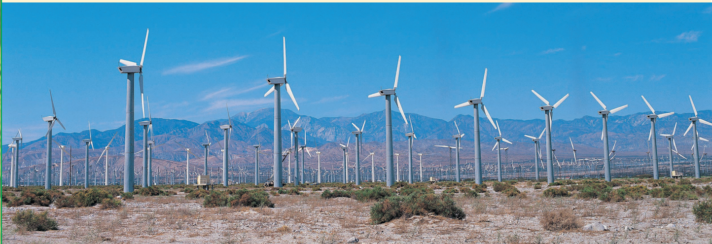
■ FIGURE 12.20 Wind-energy harvesting installation at Altamont Pass, California, which consists of over 7000 individual windmills. (©Digital Vision/PunchStock RF)
