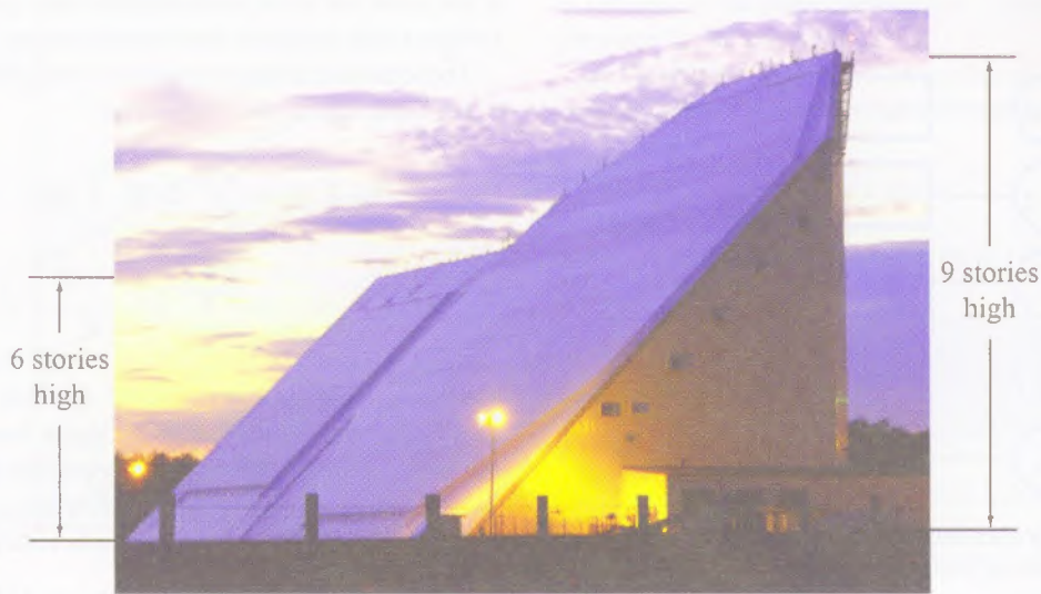
Figure 9-25: The AN/FPS-85 Phased Array Radar Facility in the Florida panhandle, near the city of Freeport. A several-mile no-fly zone surrounds the radar installation as a safety concern for electroexplosive devices, such as ejection seats and munitions, carried on military aircraft.
