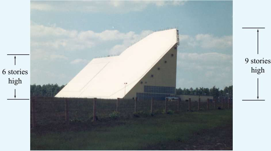
Figure 9-25 The AN/FPS-85 Phased Array Radar Facility in the Florida panhandle is near the city of Freeport. A several-mile no-fly zone surrounds the radar installation as a safety concern for electroexplosive devices, such as ejection seats and munitions that are carried on military aircraft.
